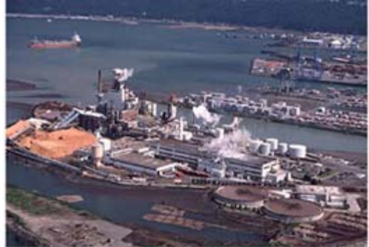
Aerial view of Simpson Tacoma Kraft Mill
